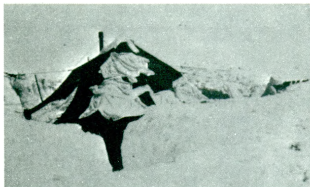
Figure 6-14. Tent dug into snow with individual firing positions.
